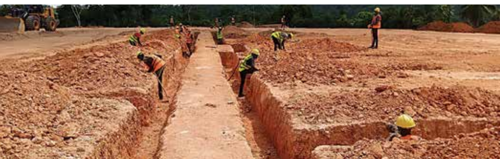
↑ Admin building foundation work
