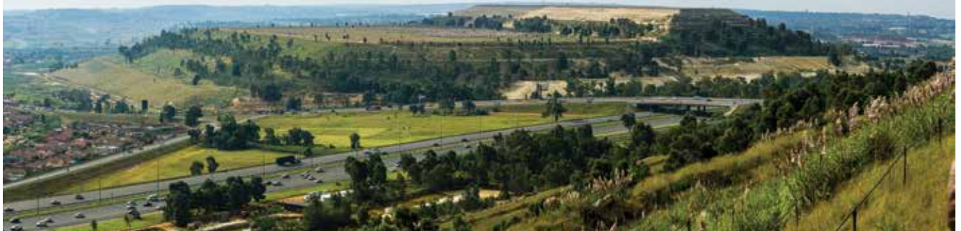
↑ Erection of windbreaks and the planting of vegetation on DRDGOLD's discontinued tailings deposition facility near Nasrec, south of Johannesburg, to contain dust pollution
