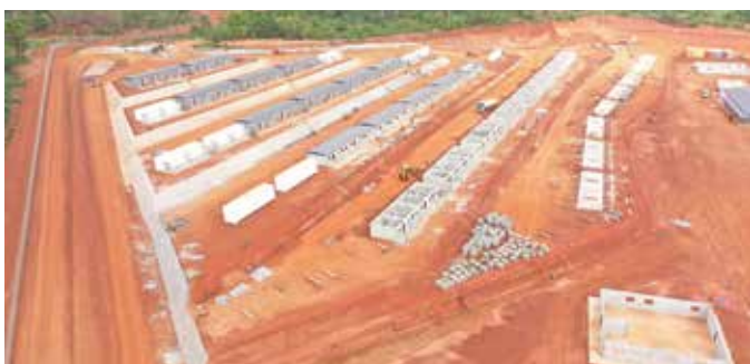
↑ Aerial view of permanent camp
