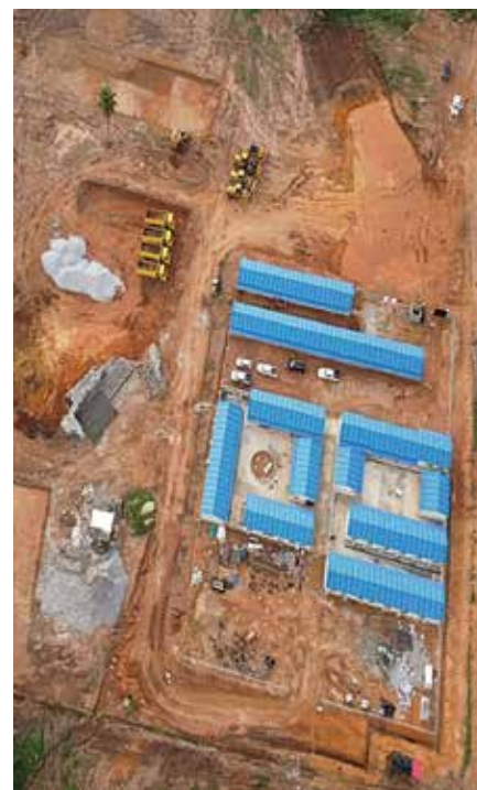
↑ Aerial picture of construction camp
