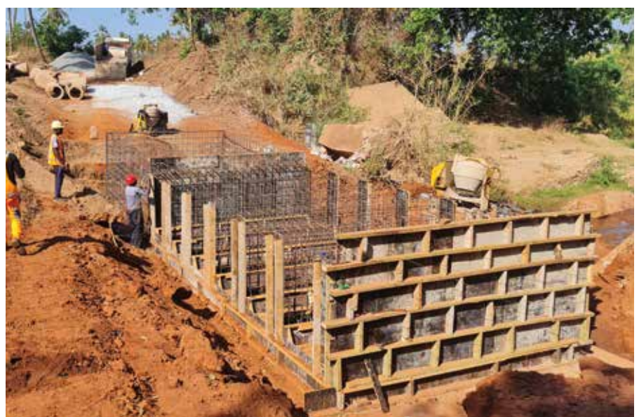
↑ Construction in full swing at Lindi Jumbo
