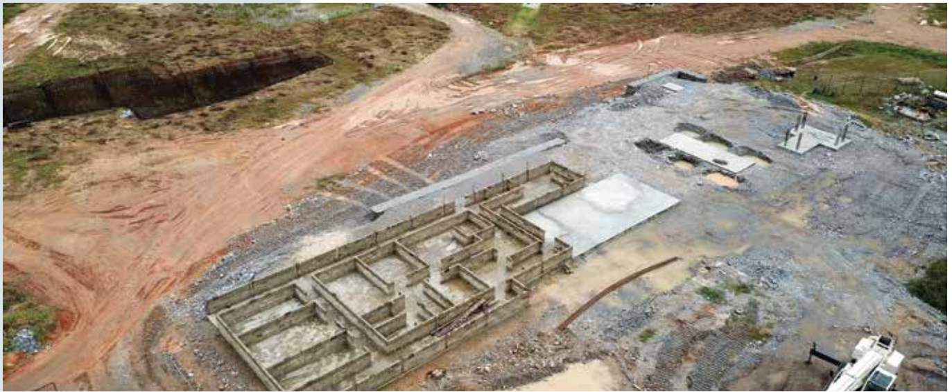
↑ 25 tph foundations with 5 tph in background
