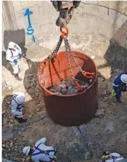
↑ Sinking activities underway
