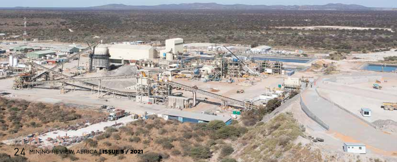
Overview of the Boseto process plant
