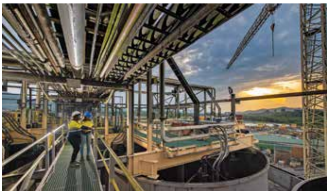
↑ By the end of March 2021, the Obuasi Redevelopment project was 97% complete
