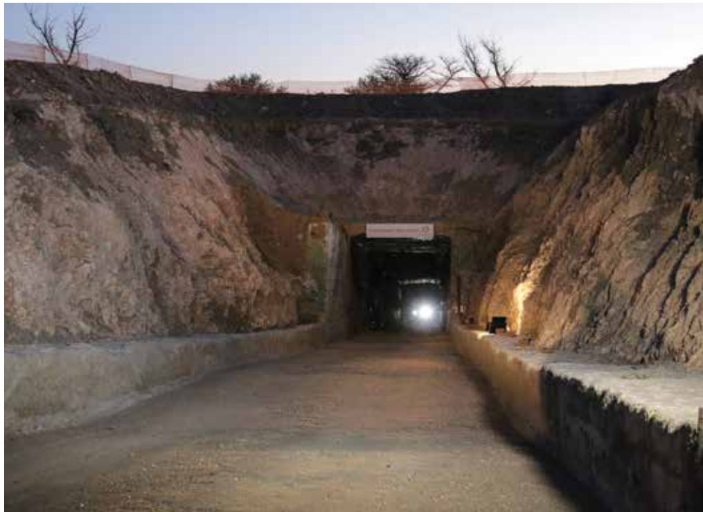
↑ Prieska copper mine decline
