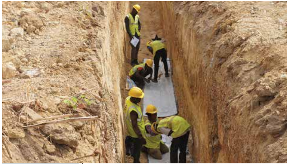
↑ Safe trenching operations at the Mint prospect
