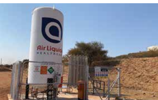
↑ The 4.5 t bulk oxygen storage tank for the supply of high flow oxygen to 56 beds in the field hospital
