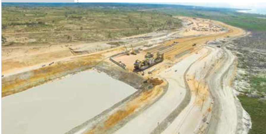
The dredge approaching its final destination at Pilivilil
