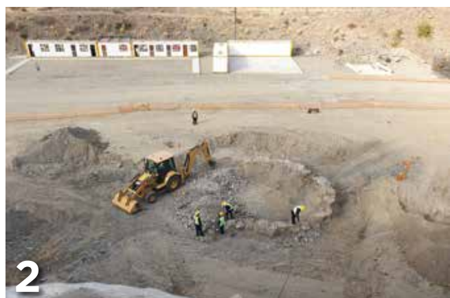
↑ Early stage works on the ventilation shaft
