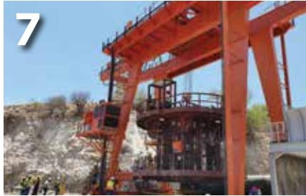
↑ Surface view of the sinking stage and supporting infrastructure
