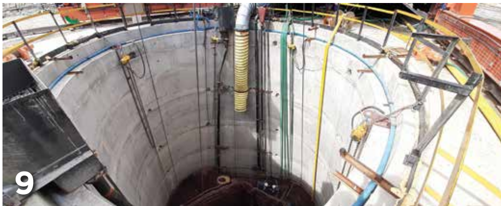
↑ View of the new ventilation shaft (as of November 2019)
