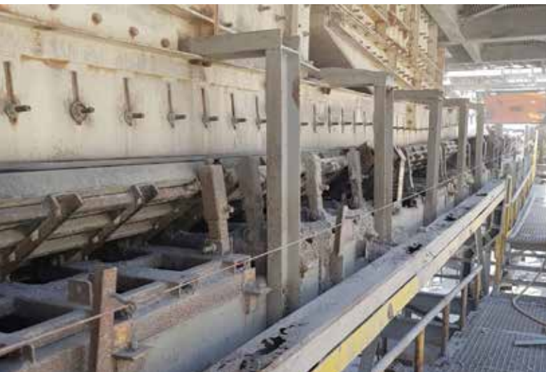
↑ Sukari gold mine: Before installation
