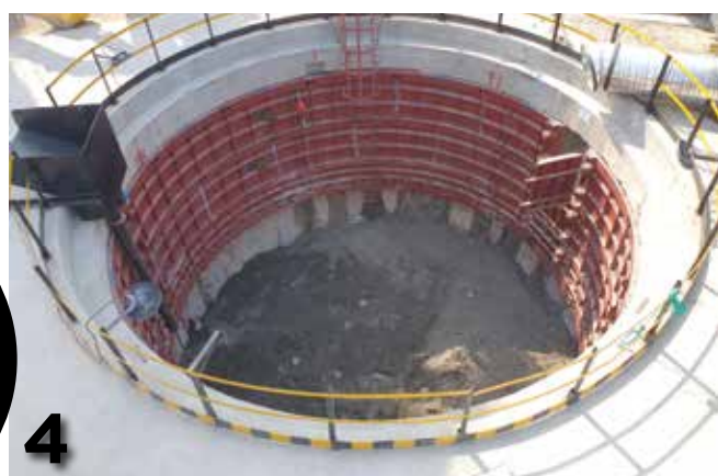
↑ Part of the four-deck stage in place
