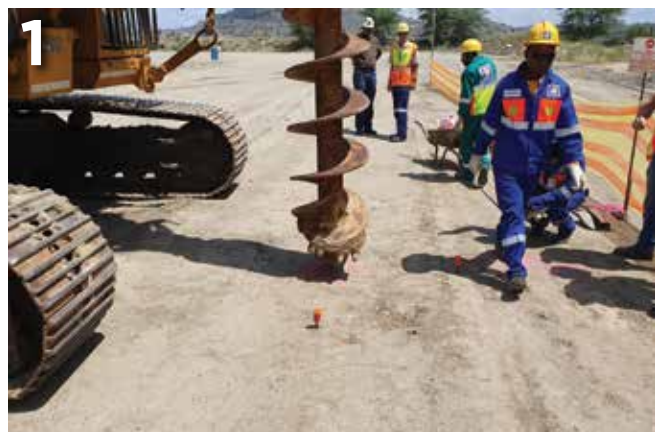
↑ Ventilation shaft ground breaking
