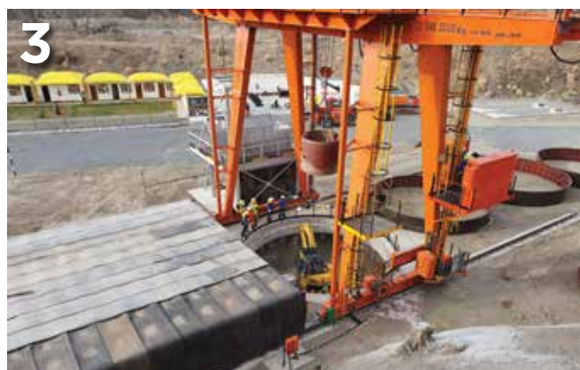
↑ Early works using a small excavator
