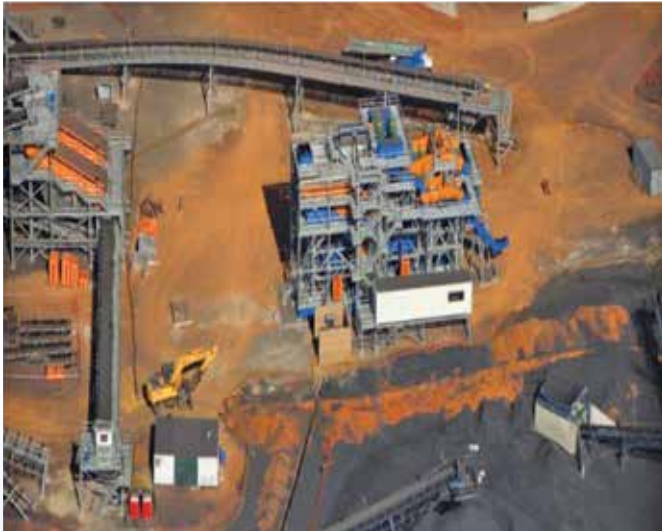
Modular Coal Processing Plants
