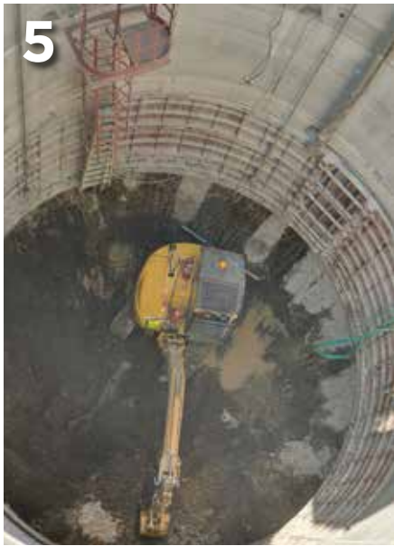
↑ The excavator underground moving blasted ore
