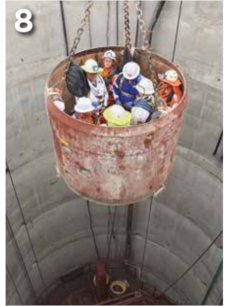
↑ Using a kibble to travel down the shaft
