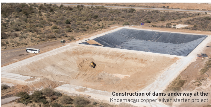
Concor Infrastructure is creating a corridor for both roads in parallel
